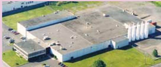
PLASTIPAK plant, Quebec, Canada.
